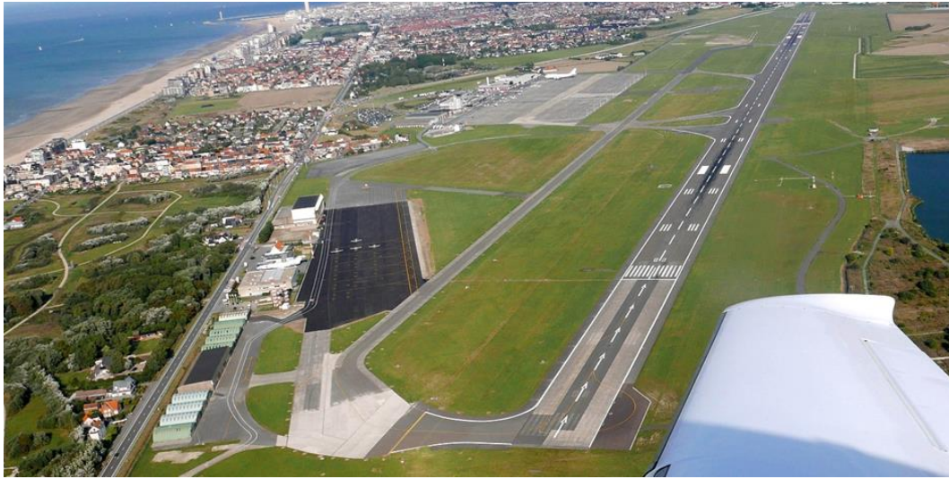
The woven geotextile was installed over 160.000m 2 of runway at Ostend-Bruges airport (Photo: © Beaulieu Technical Textiles)
