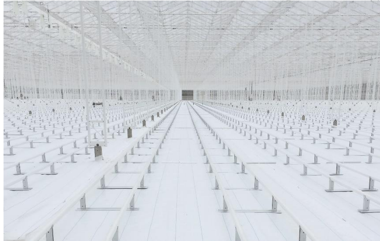
Caption: Greenhouse constructions with halogen-free flame retardant reflective groundcovers
